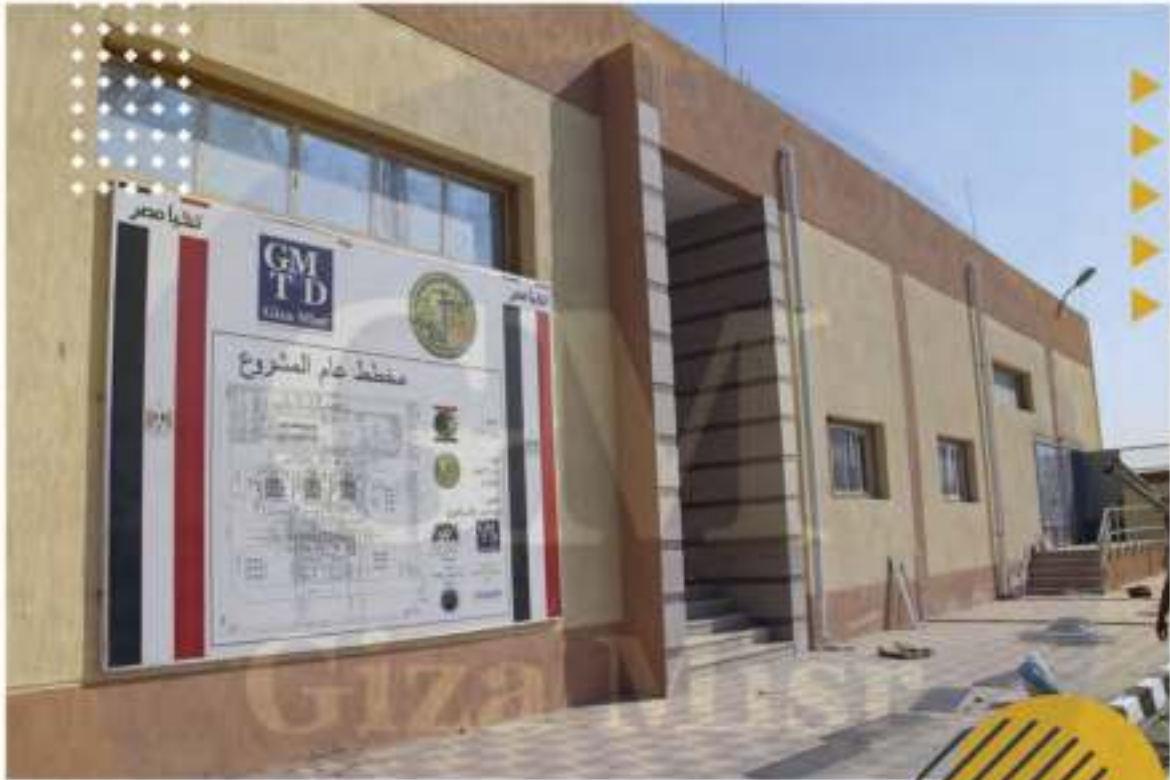
Substation West of El Shorouk 220/22/22 KV
